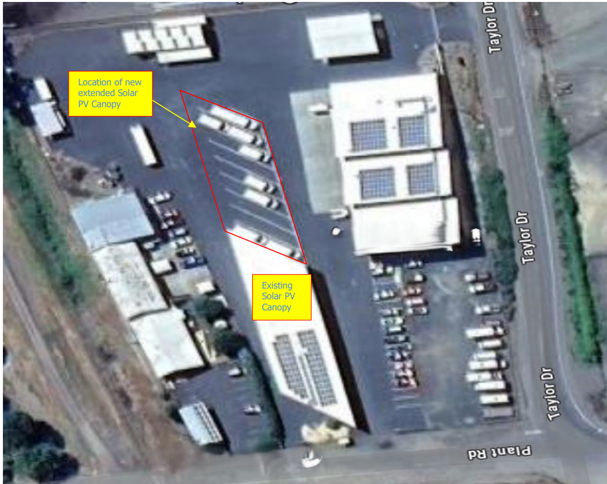
Ariel view of the Ukiah site's existing Solar PV Canopy.
